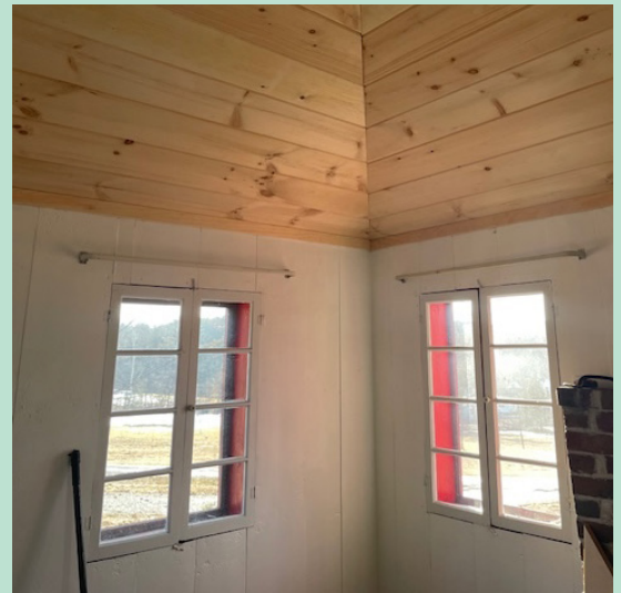
Outside Fernwood - new windows and roof (photo by Liz Ryan Cole)
